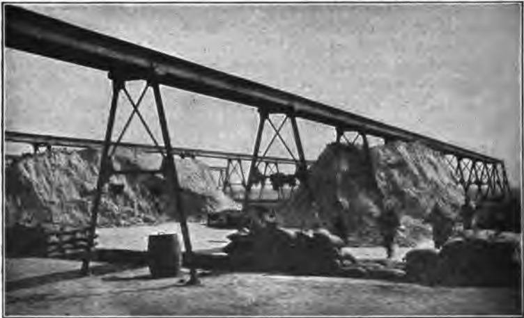
FIG. 193.—Putting nitrate into bags for shipment.
